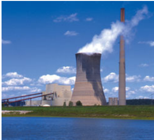
Mountaineer Plant - New Haven, WV
