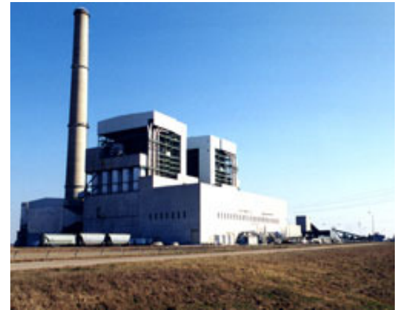
Northeastern Plant - Oologah, OK
