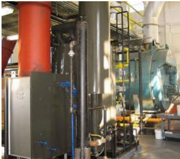
Ethicon Cornelia, GA Boiler Upgrade
