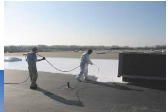
Healthcare Systems Memphis, TN Cool Roof Coating
